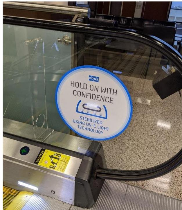
**Figure 3.3** Example of UV-Light Disinfection of Escalator Handrail
